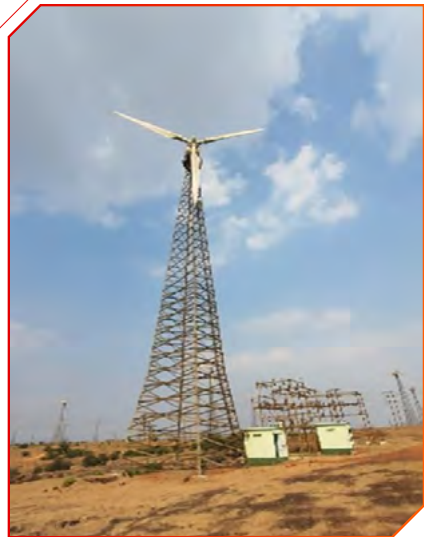
350kW WTG at Vankusawade Site, Satara, Maharashtra
